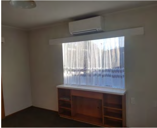
Lounge – Repaint & Heatpump
